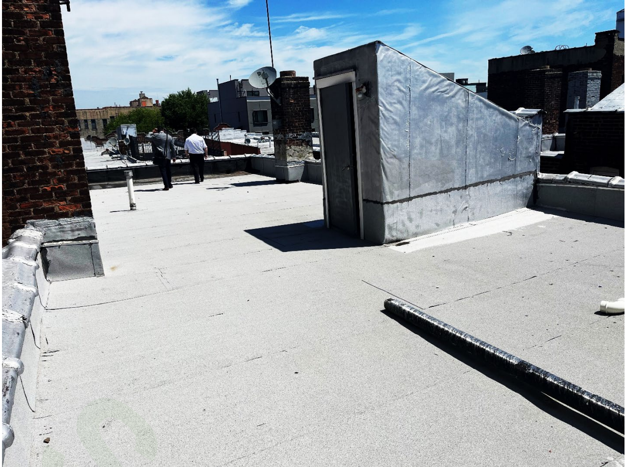
Figure 22 - View of [REDACTED] roof
